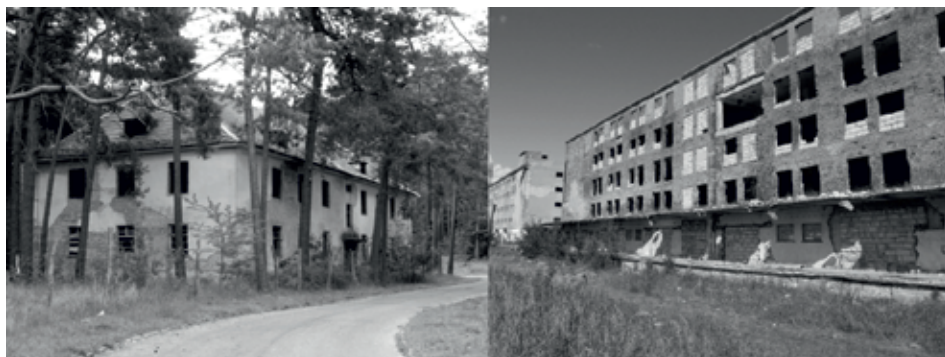
Fig. 2. Dilapidated residential dwellings and warehouses at Borne Sulinowo
